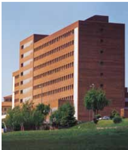
Hospital General de Vic
